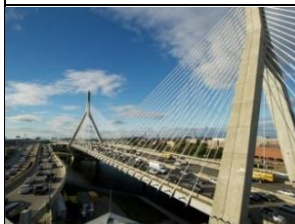
Leonard Zakim Bunker Hill Memorial Bridge, Boston
