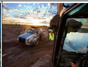
Tres Rios Ecosystem Restoration and Flood Control Project, Phoenix
