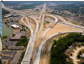
Interstate 465 Reconstruction, Indiana
