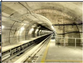
Washington Dulles International Airport Tunnel
